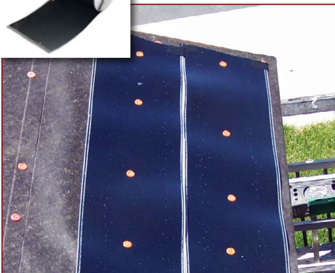
ProLine low-voltage roof heating element being installed.
