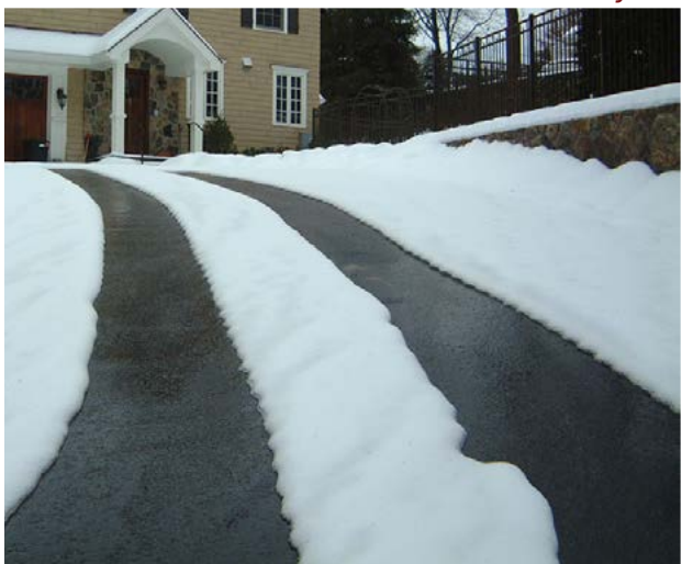
Heated tire tracks in asphalt driveway.
