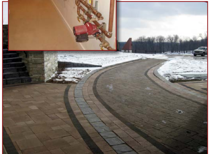
ProLine Radiant hydronic snow melting system's mechanical / boiler room (left) and photo of system installed under pavers (below).
