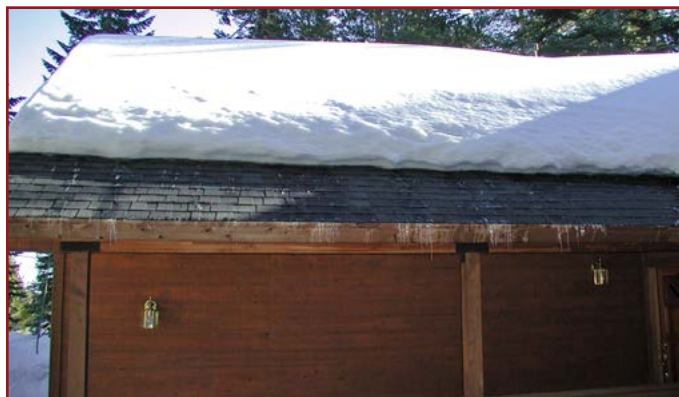
Eliminate ice dams by heating roof edges.
