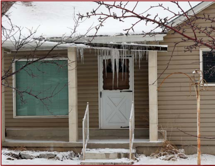
Pictured above is an example of gutter damage caused by heavy ice buildup.
