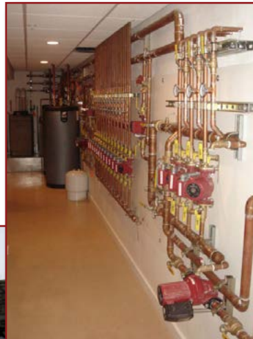
ProLine Radiant hydronic snow melting system's mechanical / boiler room (left) and photo of system installed under pavers (below).
