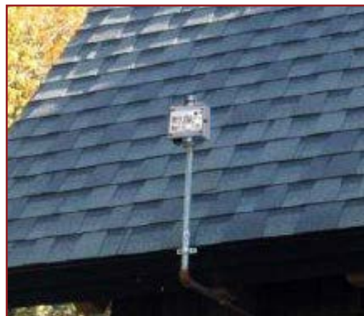
ProLine radiant snow melting system with aerial-mount snow sensor installed at roof's edge.
